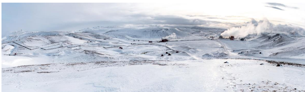
Fig. 5. The Krafla geothermal power plant close to the Krafla Volcano and the lake Mývatn, Iceland (©Mauro Passarella, 2019)
